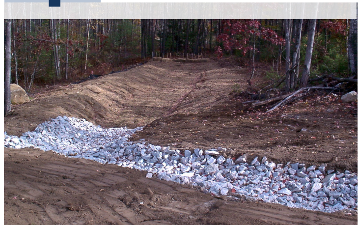
Riprap installation
