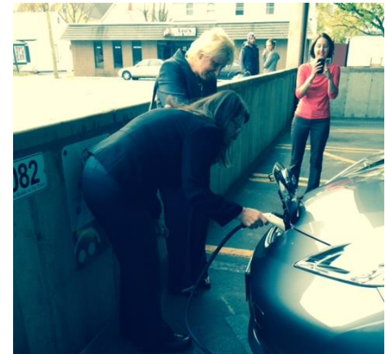
The City of Nashua recently partnered with Public Service of NH to install an electric vehicle charging station (PSNH)
